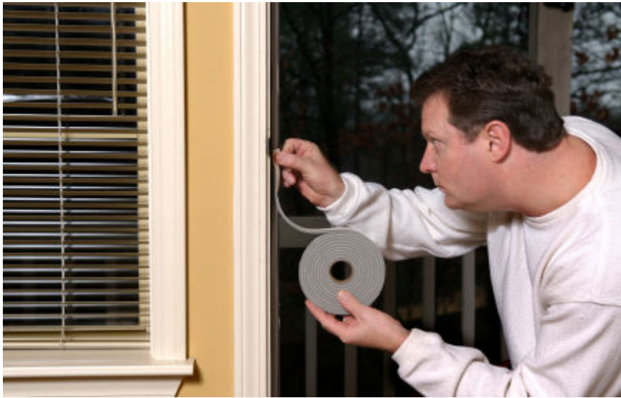
Most older homes have cracks around windows and doors that allow a significant amount of heat to seep out.
